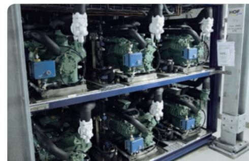
Fig.: Module structure of six compressors
